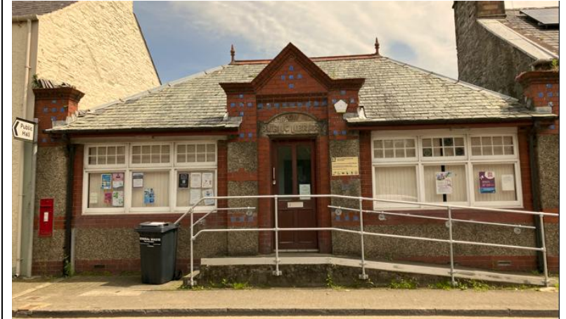
The early 20 th century library on St. John's Street, brick built with a distinct symmetrical front elevation with ceramic brick and terracotta detailing and a stone lintel with inscription and date above central entrance door.
