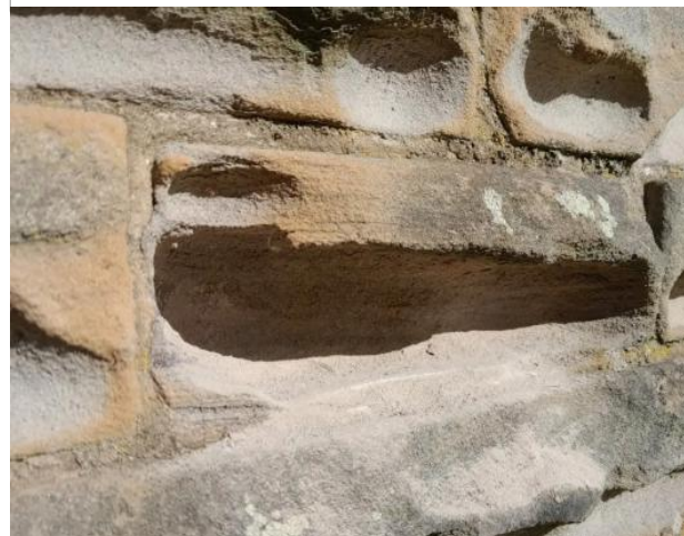
Damaging use of cement render on whinstone and sandstone rubble elevation now defacing the sandstone.
