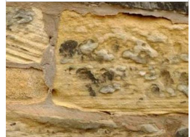
Cement pointing damage to sandstone
