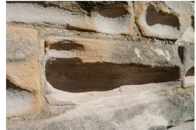
Cement pointing damage to sandstone
