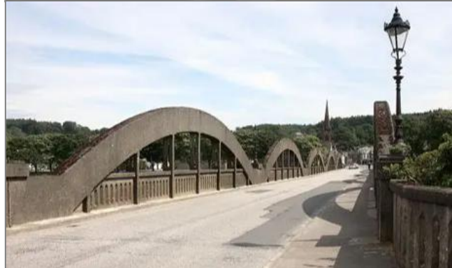
Top: Former bowstring iron bridge over the Dee from 1868 and Below: B Listed 1926 concrete bowstring bridge over the Dee.
