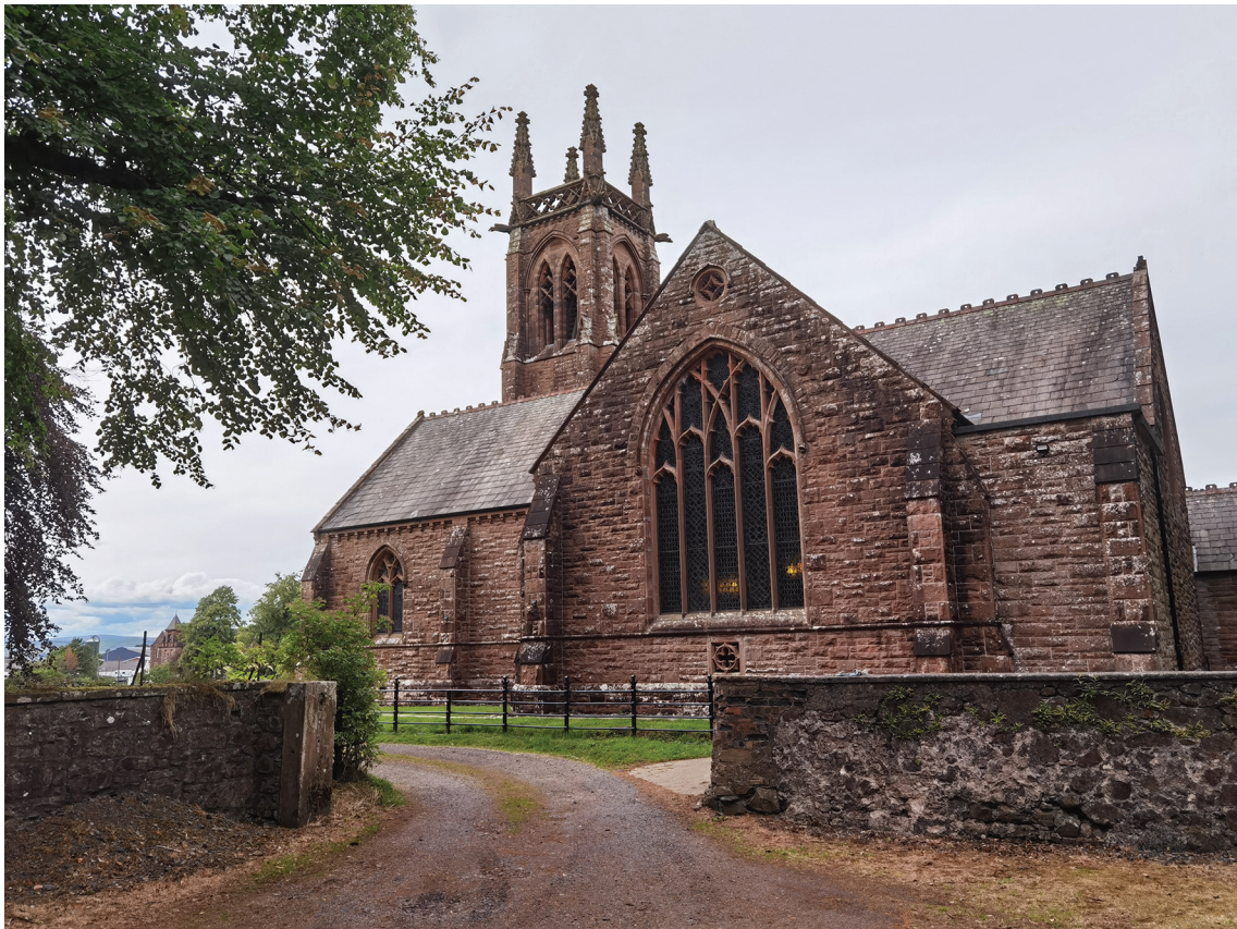
Fig 3 Closeburn Parish Church
