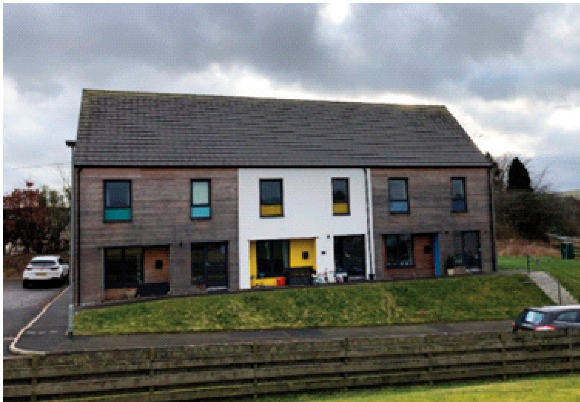
Fig 8 Closeburn Passivhaus Homes
