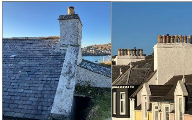
Natural slate roof, stone ridge capping and skew stone and right, a selection of chimneys, building heights and dormers creating a varied roovescape
