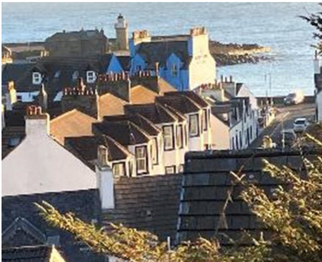
Regular roovescape and dormers of two terraces along the street named Blair Terrace
