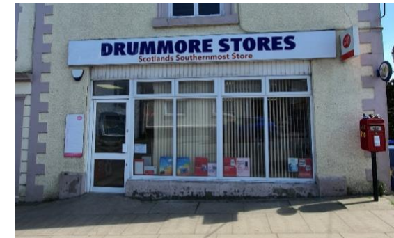
Drummore Village Shop and Post Office
