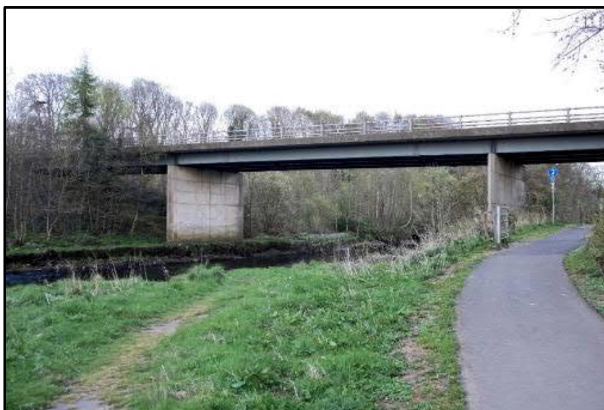
Figure 3-10 - View Beneath A75T Bridge Looking Downstream
