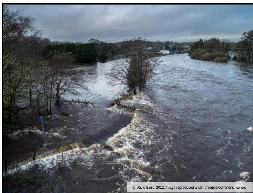
Figure 3-11 - View Beneath A75T Bridge Looking Upstream from Bridge Deck During Flood
